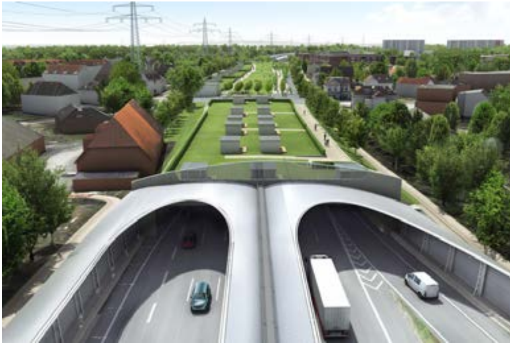
Proposed Decking of A7 highway, Hamburg, Germany
